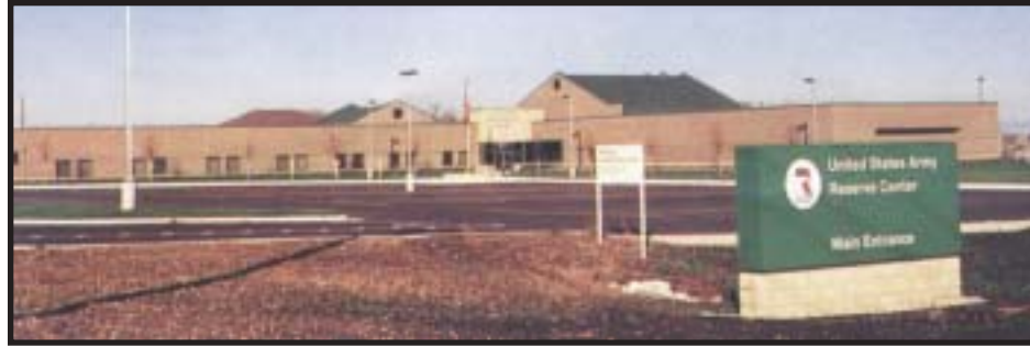
U.S. Army Reserve Center U.S. Army Corps of Engineers Sturtevant, WI Thomas Mason Painting Contractor
