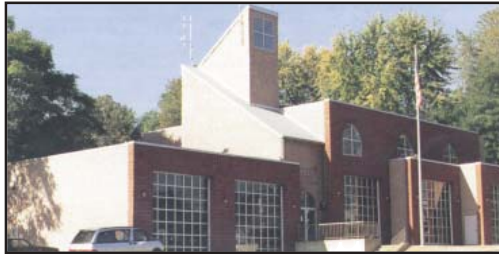
Fire Station - Pleasant Hill, PA Contractor - Tri-State Waterproofing Photo credit: T.E. Auel
