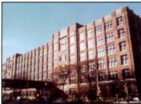
Milwaukee Area Technical College Architect: Staff Contractor: Wisconsin Restoration-Garon Contractors Specifications included brick cleaning and waterproofing with Diedrich Chemicals
